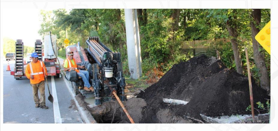
Picture of a directional bore machine that will plow in innerduct and fiber is blown through that. We put in that innerduct and fiber.
